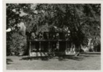
McAlpin House (demolished) (MS 0061-24-13-001)
