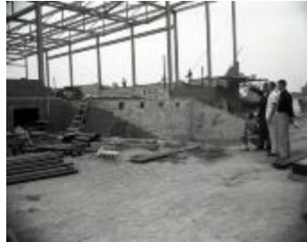
Gym construction (MS_0045-249)
