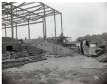
Gym construction and onlookers (MS_0045-250)
