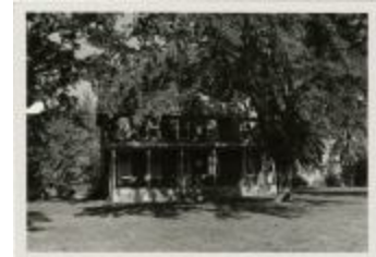
McAlpin House (demolished) (MS 0061-24-13-001)
