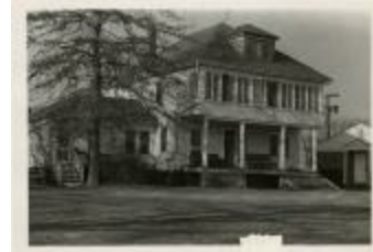
Richmond House (demolished) (MS 0061-25-03-001)
