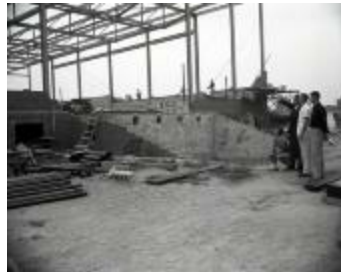
Gym construction (MS_0045-249)
