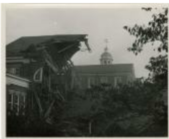
Demolition of Cain Gym (MS 0061-22-12-001)
