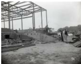
Gym construction and onlookers (MS_0045-250)
