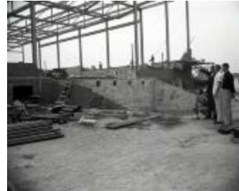
Gym construction (MS_0045-249)
