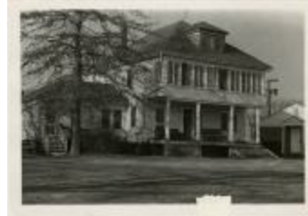
Richmond House (demolished) (MS 0061-25-03-001)
