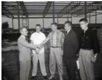
Group of men in front of gym construction (MS_0045-251)
