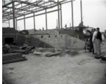
Gym construction (MS_0045-249)
