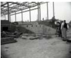
Gym construction (MS_0045-249)
