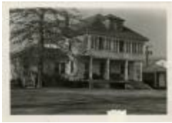
Richmond House (demolished) (MS 0061-25-03-001)
