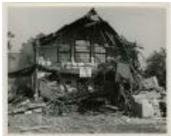
Demolition of Cain Gym (MS 0061-22-12-003)
