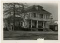
Richmond House (demolished) (MS 0061-25-03-001)
