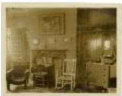
Typical Room in Reid Hall (MS 0061-24-19-012)
