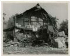
Demolition of Cain Gym (MS 0061-22-12-003)
