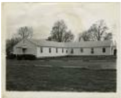
G.I. dorms (demolished) (MS 0061-23-16-007)
