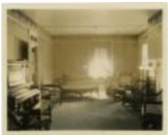
Social Room in Reid Hall (MS 0061-24-19-011)
