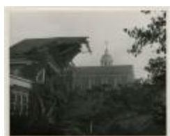
Demolition of Cain Gym (MS 0061-22-12-001)
