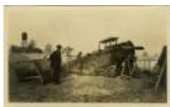
Biplane repairs (MS 0083-01-01-003)
