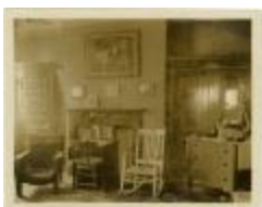
Typical Room in Reid Hall (MS 0061-24-19-012)
