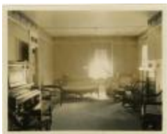
Social Room in Reid Hall (MS 0061-24-19-011)
