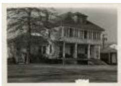
Richmond House (demolished) (MS 0061-25-03-001)
