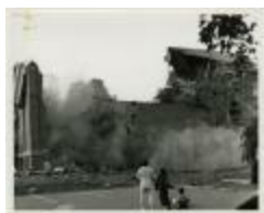
Demolition of Cain Gym (MS 0061-22-12-004)
