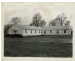
G.I. dorms (demolished) (MS 0061-23-16-007)
