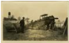
Biplane repairs (MS 0083-01-01-003)
