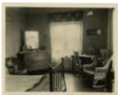
Room in Reid Hall (MS 0061-24-19-010)
