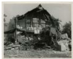
Demolition of Cain Gym (MS 0061-22-12-003)
