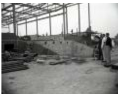
Gym construction (MS_0045-249)
