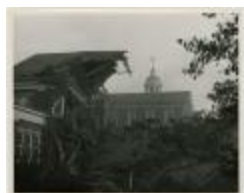
Demolition of Cain Gym (MS 0061-22-12-001)
