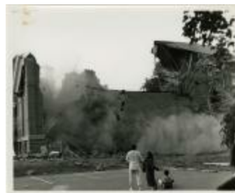
Demolition of Cain Gym (MS 0061-22-12-004)
