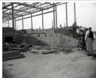
Gym construction (MS_0045-249)
