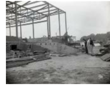
Gym construction and onlookers (MS_0045-250)
