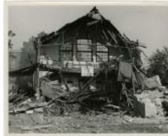
Demolition of Cain Gym (MS 0061-22-12-003)
