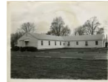
G.I. dorms (demolished) (MS 0061-23-16-007)
