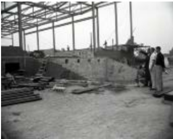
Gym construction (MS_0045-249)
