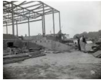
Gym construction and onlookers (MS_0045-250)
