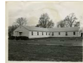
G.I. dorms (demolished) (MS 0061-23-16-007)
