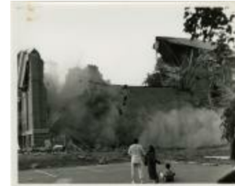
Demolition of Cain Gym (MS 0061-22-12-004)
