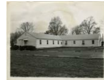
G.I. dorms (demolished) (MS 0061-23-16-007)
