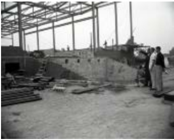
Gym construction (MS_0045-249)
