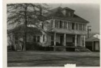
Richmond House (demolished) (MS 0061-25-03-001)
