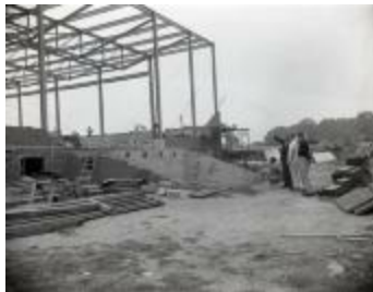
Gym construction and onlookers (MS_0045-250)
