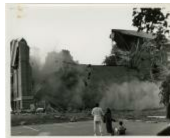
Demolition of Cain Gym (MS 0061-22-12-004)
